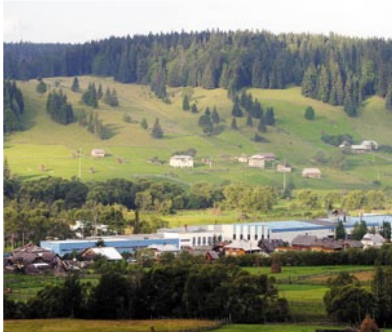
Dorna mineral water bottling plant located in the foothills of the Carpathians at Vatra Dornei, Romania
