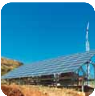
Pilot "Green" Base Station
