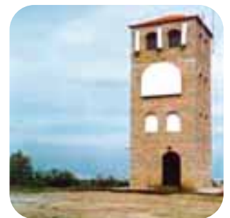
Base Station special construction
