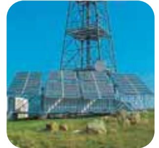
Photovoltaic system in Base Station
