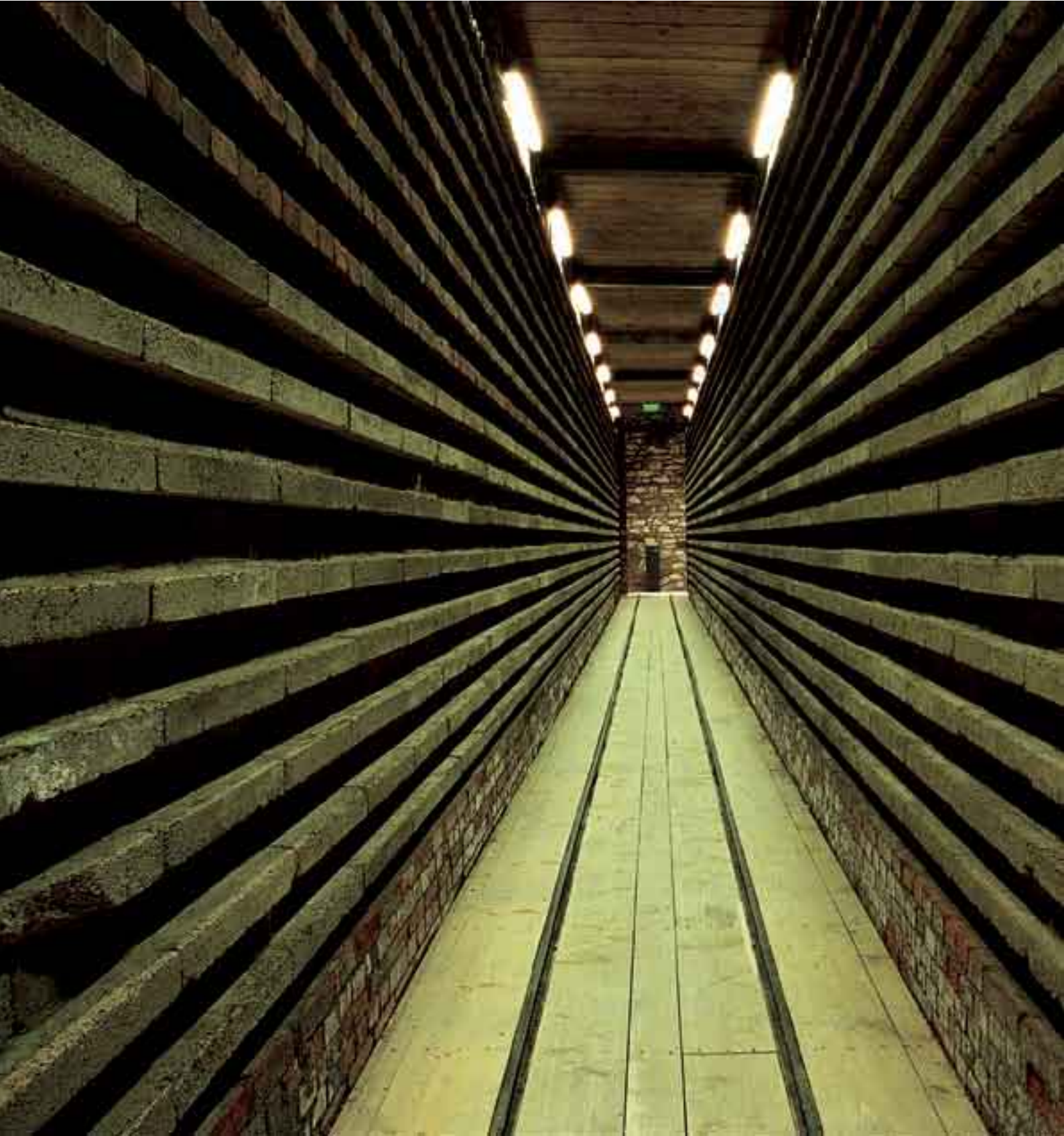
Rooftile and Brickworks Museum N. & S. Tsalapatas. Interior view of the driers.
