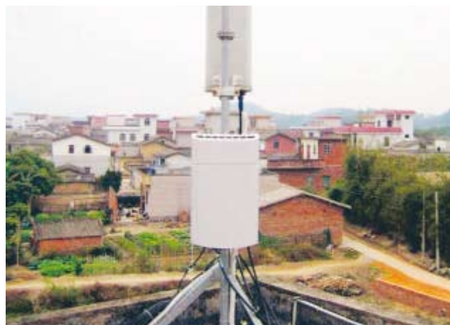
Ericsson's main remote, tower-mounted radio base stations cut energy consumption compared to those located on the ground.
