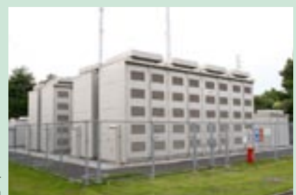
NAS battery power storage system
