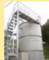
"Bio Attack," designed to decompose wastewater using microorganisms
