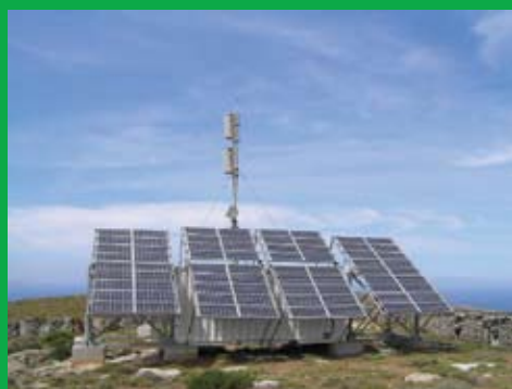
Photovoltaic system in Base Station
