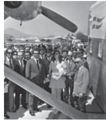
Construction of Milos airport with S&B's financial and technical assistance.
