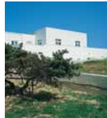
Construction of the Pollonia Cultural Center on Milos.
