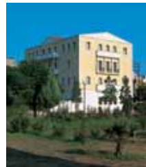
Construction of the Itea Cultural Center.
