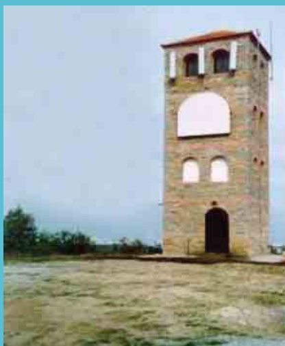
Base Station special construction
