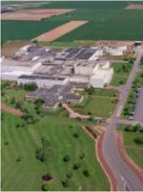
Each manufacturing facility, such as this one in Arras, France, must identify, track and report on key environmental parameters.
