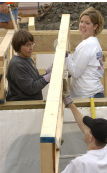
A majority of employees are active volunteers. Habitat for Humanity brings volunteers together to build homes for low-income buyers.
