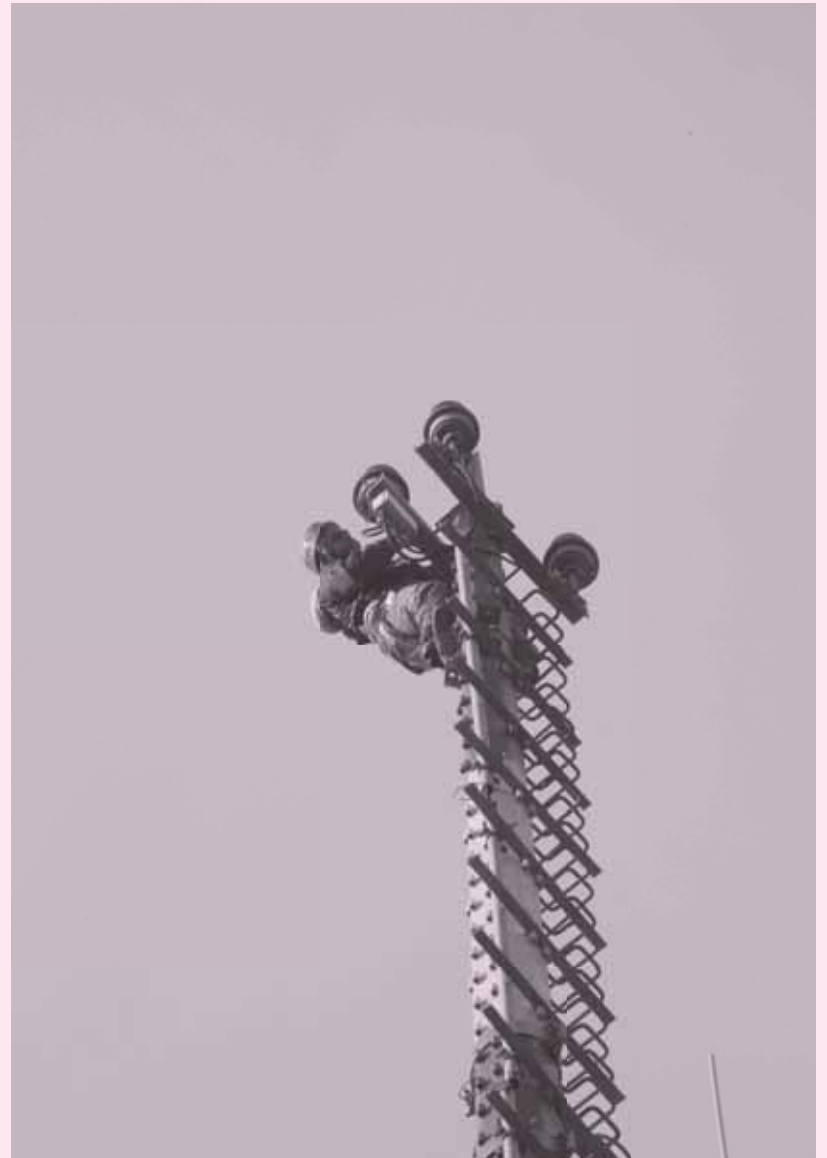
OTE lineman on the job.
