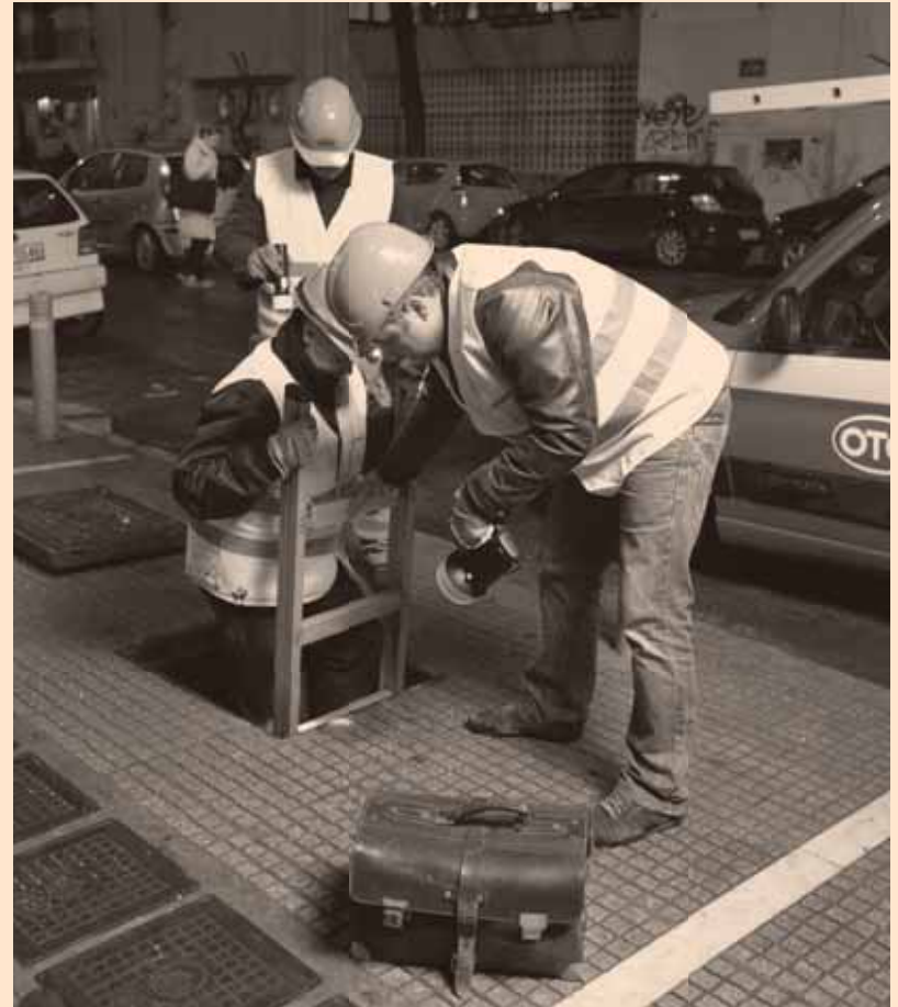
An OTE repair crew, making repairs at the Center of Athens.
