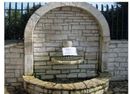
A tap with special photocell for controlled use of water by the nearby residents, is in place at Aegio Plant.
