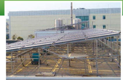
Solar panels to heat boiler water were installed at two of our plants in China.
