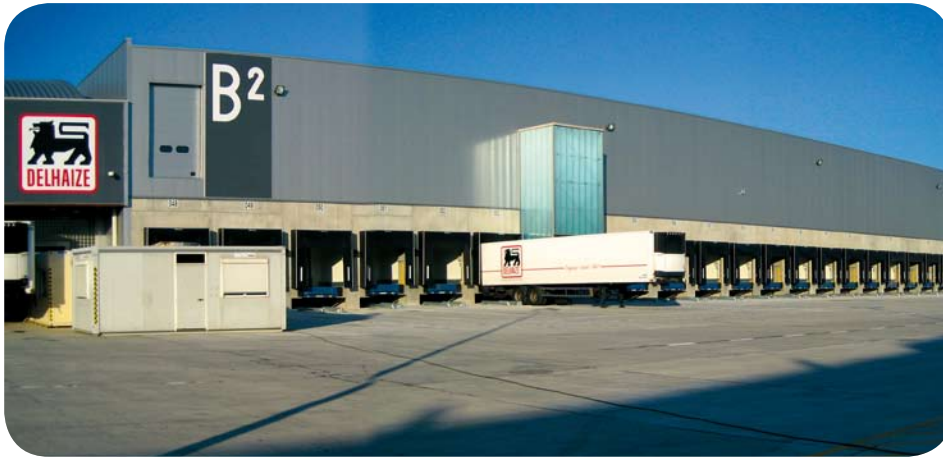
Delhaize Belgium's new distribution center uses a CO 2 refrigeration system
