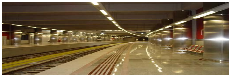
View Metro Station: Ag. Antonios
