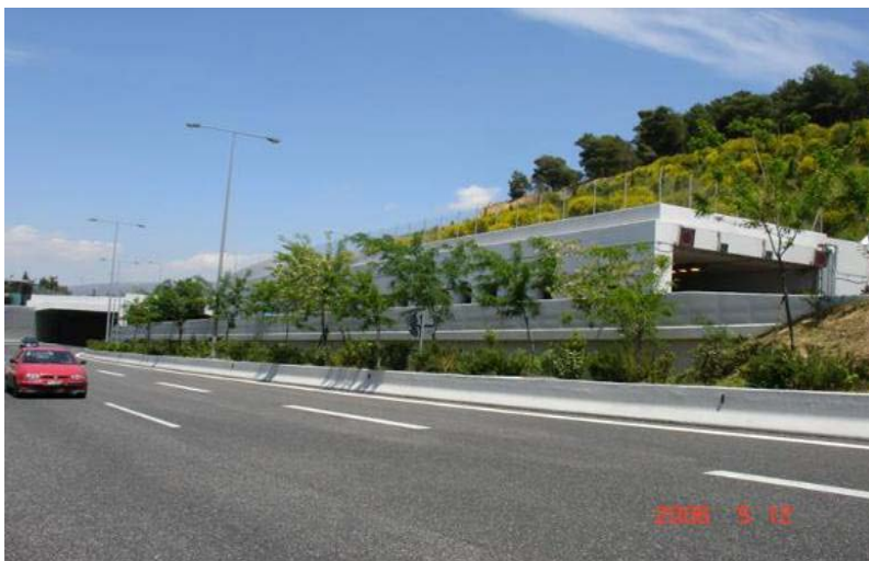
View of west peripheral Ymmitos Highway
