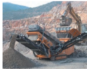
RECYCLING UNIT AT HALKIS
