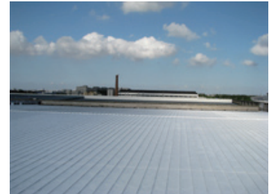
Insulating paint on the roof of Shanghai Suoguang Visual Products
