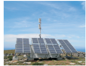
Photovoltaic System in Base Station
