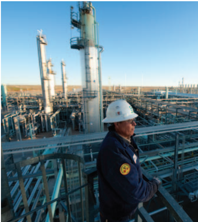
Seminole Gas Processing Plant, Texas
