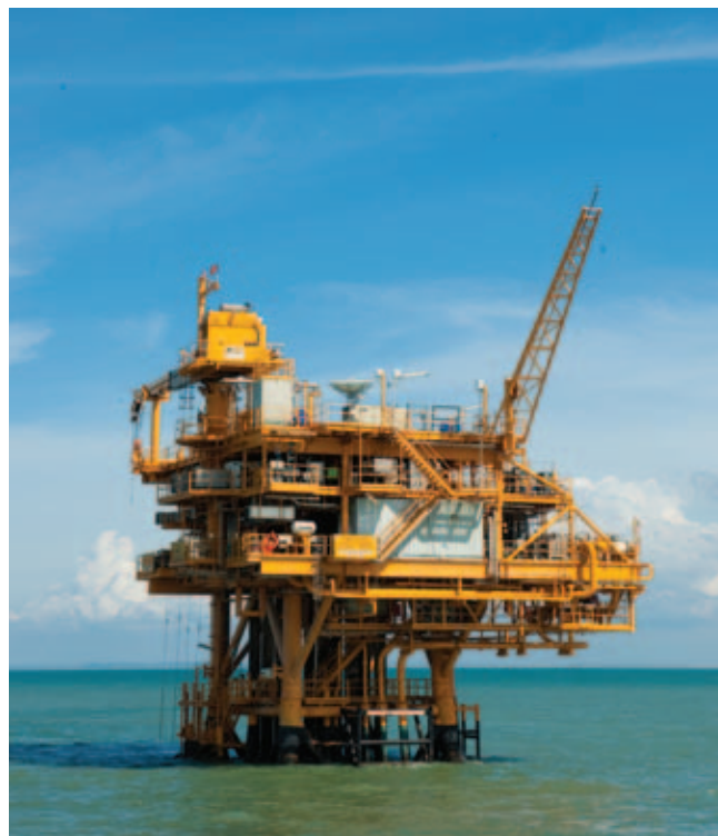
Wellhead Platform A, Offshore Pangkah, Indonesia
