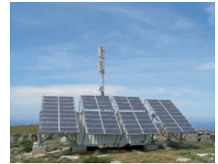
Photovoltaic System in Base Station
