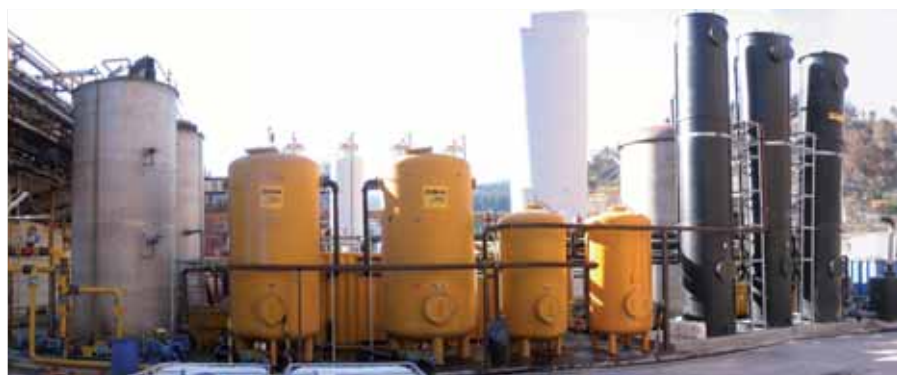
Units to treat contaminated underground water at Bussi sul Tirino (Italy)
