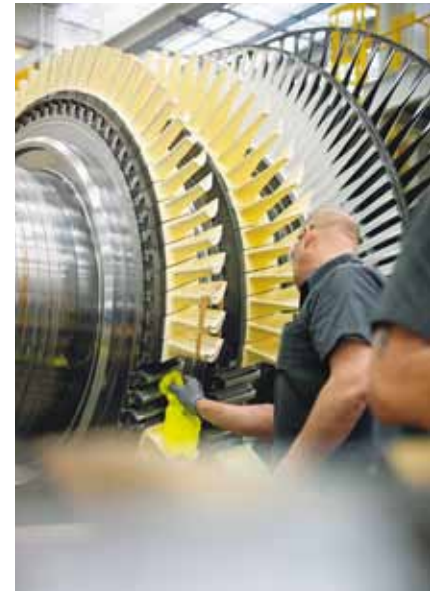
ABOVE – Our state-of-the-art combined cycle power plants make a major contribution to protecting the environment and climate: A power plant equipped with a 570-MW 8000H gas turbine can reduce CO 2 emissions by 700,000 tons a year compared with the average for all plants worldwide.
