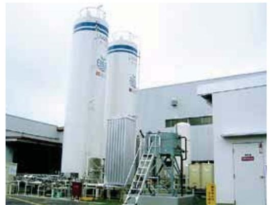
Exterior of the cogeneration system: Liquefied natural gas tank (left) and gas engine power generator building (right)
