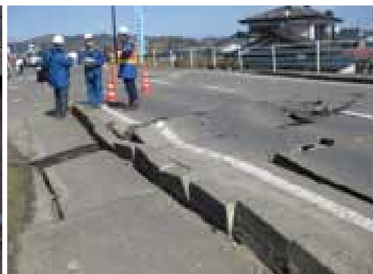
A road section where a cable pipe/culvert crossing earth fill has subsided. A trunk line cable is buried beneath this section.
