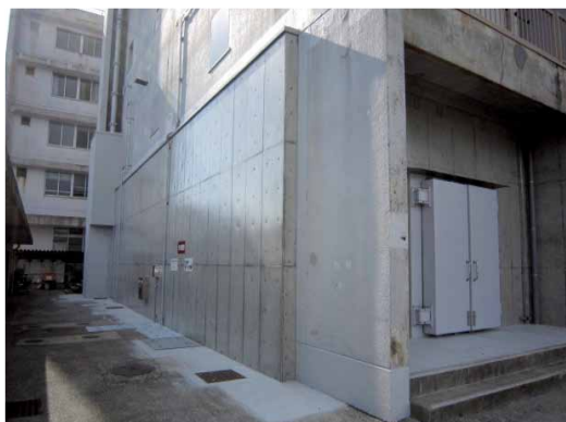
Walls and doors of communications buildings have been reinforced and made more airtight as a flood defense measure
