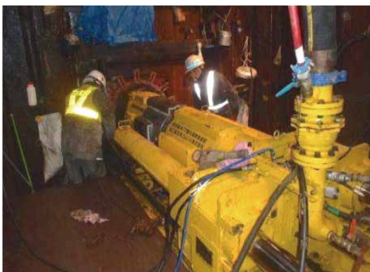
Burrowing below rivers to lay trunk line cables
