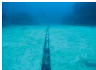
Laying submarine cables to avoid coral reefs
