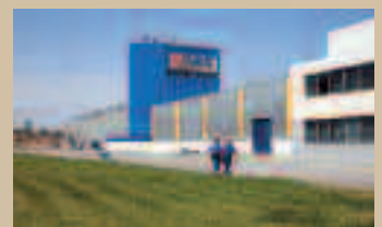
HELLENIC CABLES, Livadia, Greece
