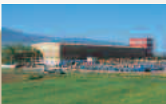
HELLENIC CABLES, Thiva, Greece
