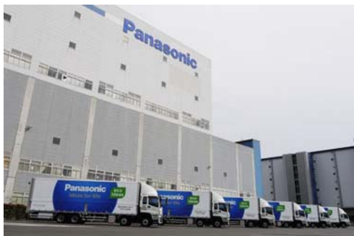
Large CNG-powered vehicles owned by Panasonic
