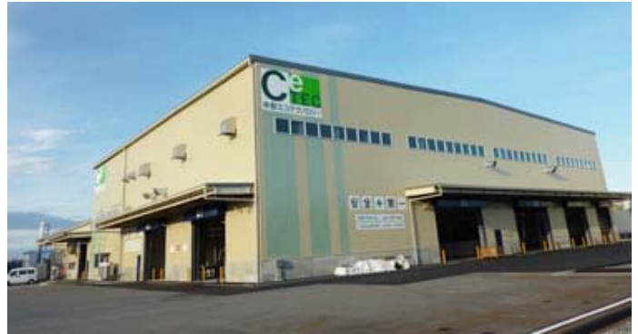
New plant at CETEC
