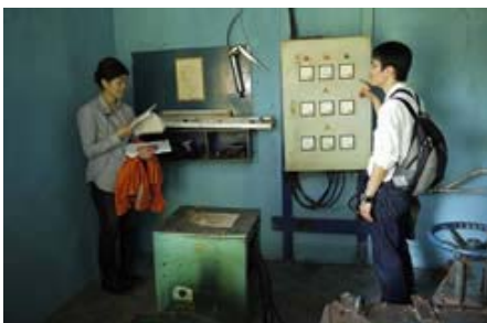
The two Panasonic employees inspect the power generation system.
