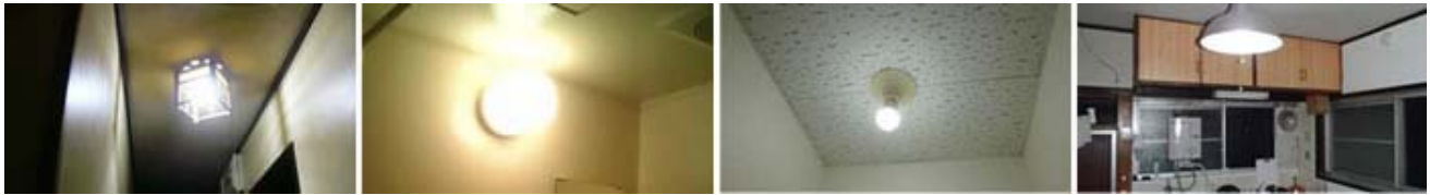
Donated LED lights being installed
