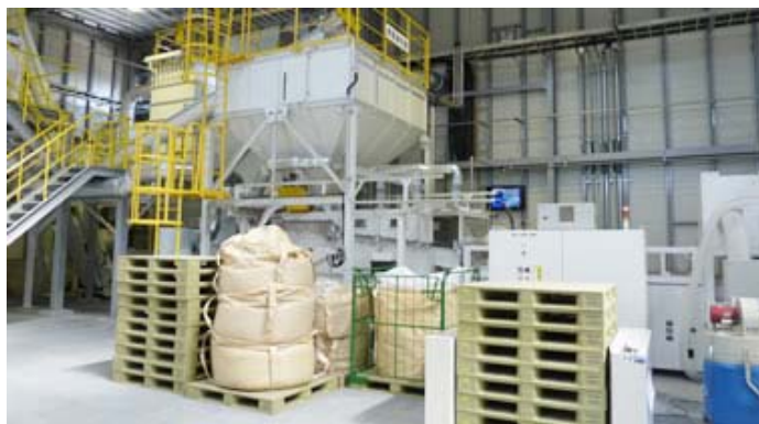
High-precision resin sorting system additionally installed at PETECK
