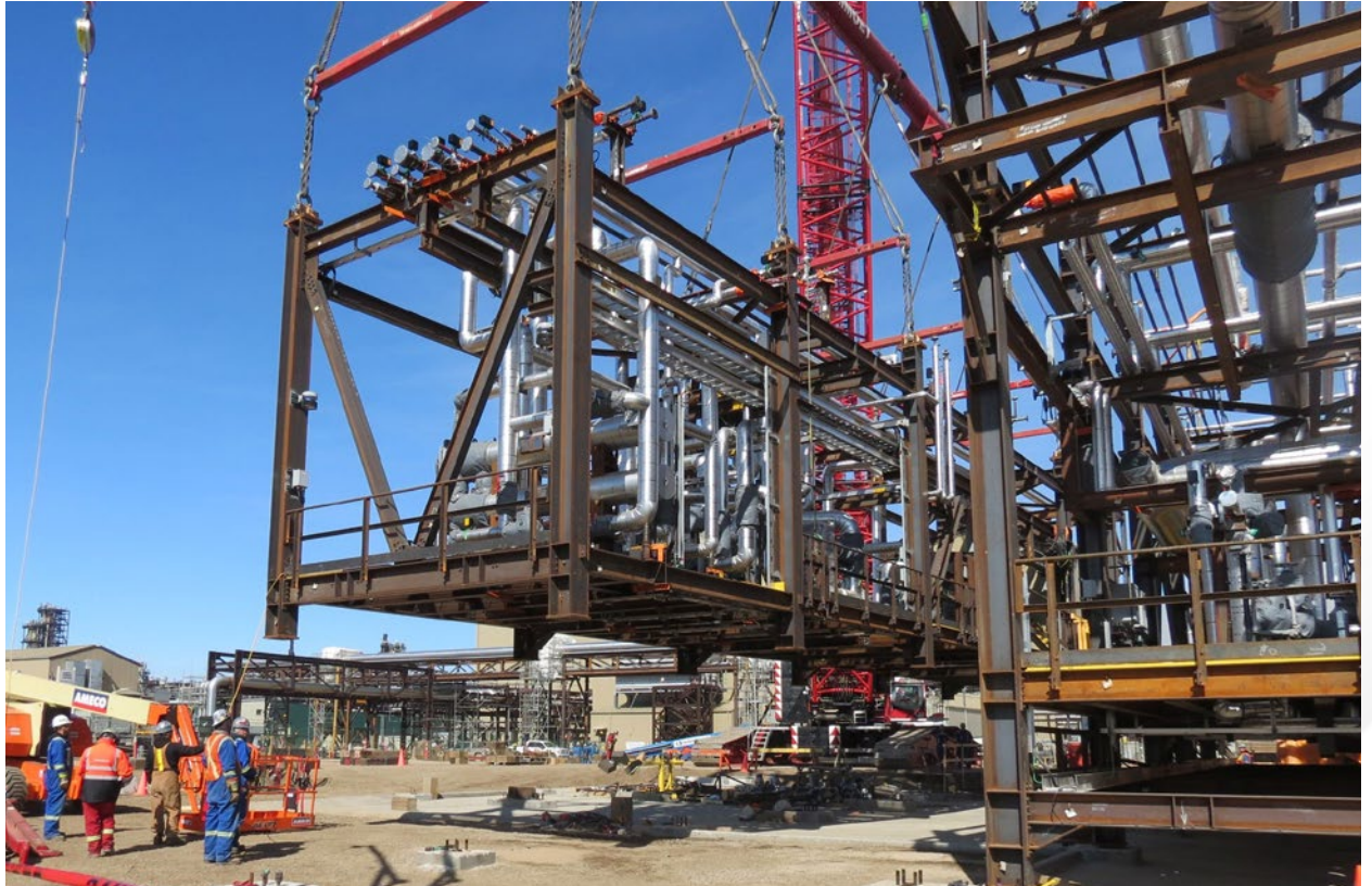
Modular Units on Quest Carbon Capture and Storage Project, Edmonton, Alberta, Canada.
