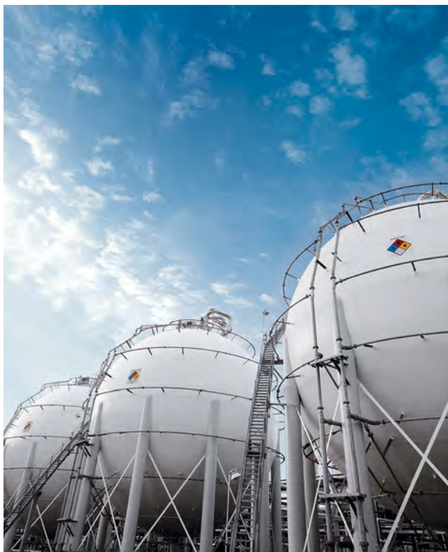
The Natrium processing and fractionation facility in Marshall County, W.Va., entered service in 2013. The plant, which was contributed to the Blue Racer joint venture, helps natural gas producers in the Appalachian Basin by extracting and separating natural gas liquids from the gas stream for transportation across interstate pipelines.
