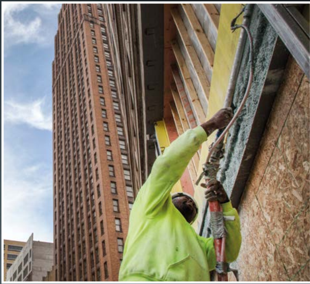
Photo above: Alongside CDFIs, traditional community development banking efforts are providing critical capital to fuel Detroit's recovery. Here, a worker sprays fireproofing on a new development at 1145 Griswold, in the long-neglected Capitol Park in the heart of downtown. Projects like this and the Scott Building, which will break ground in early 2016, are visible signs of Detroit's revitalization.
