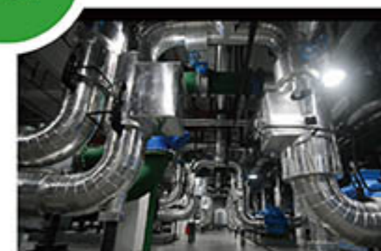
Water cooling system in ICBC Data Center (Shanghai)
