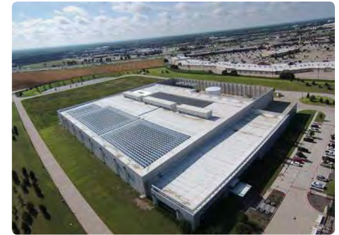
Cisco’s Allen, Texas, Data Center Solar Project
