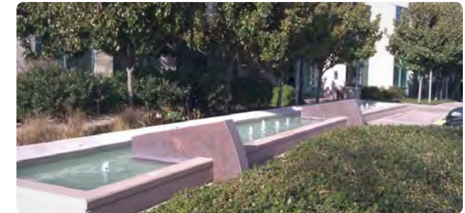
San Jose, California, Decorative Fountain (Before)
