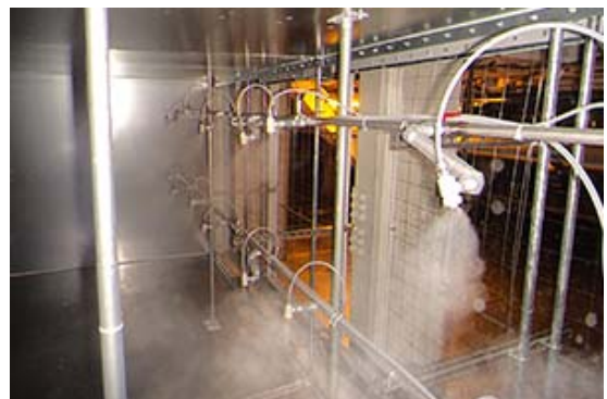
The two-fluid humidification system releases mist.
