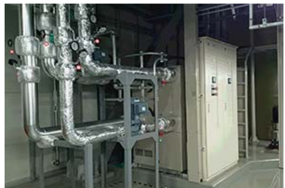
A highly efficient heat recovery system was installed in the pure water room
