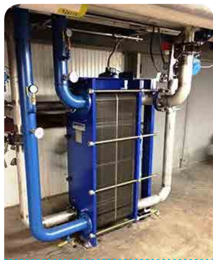
△ Duplex hot water heat recovery exchanger in Cedar Rapids, Iowa.
