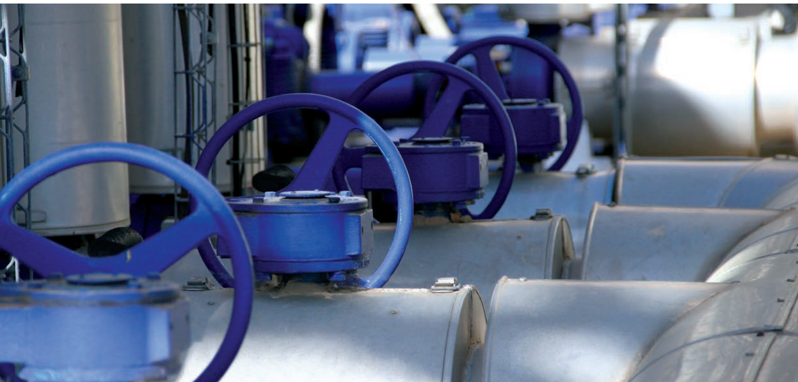
Water system, Rousset, France
